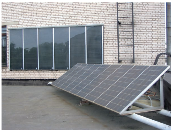
Figure 4. Overview of solar water heating and photoelectric stations, ISEU.
